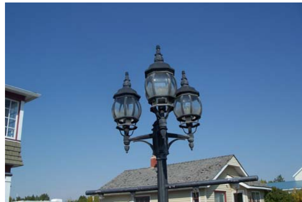
Prohibited decorative luminaire (Unshielded, exposed lamp)
